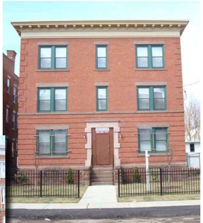
These apartment buildings have been rehabilitated as duplexes. Left: 19 Edgewood Street. Right: 29 Edgewood Street.
