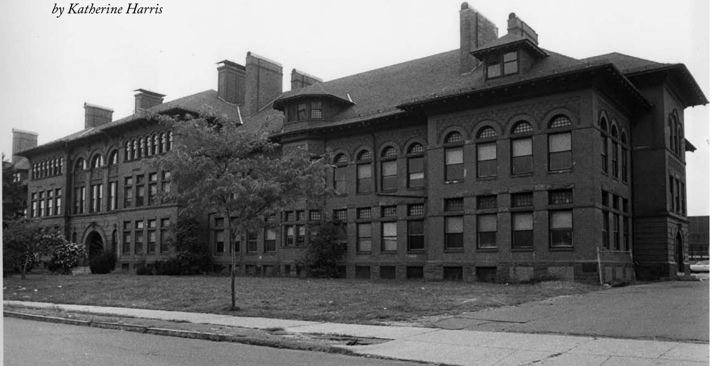
Northwest District School, circa 1978. Now mostly demolished.
