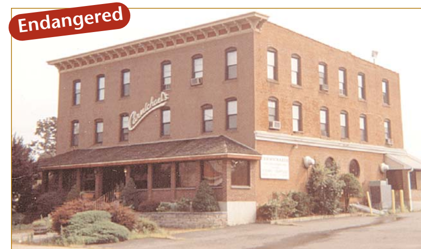
The former Carmichael's Restaurant at 682 Wethersfield Avenue and three other buildings are slated for demolition in order to build a shopping plaza anchored by a CVS pharmacy. Photo: Tomas J. Nenortas
