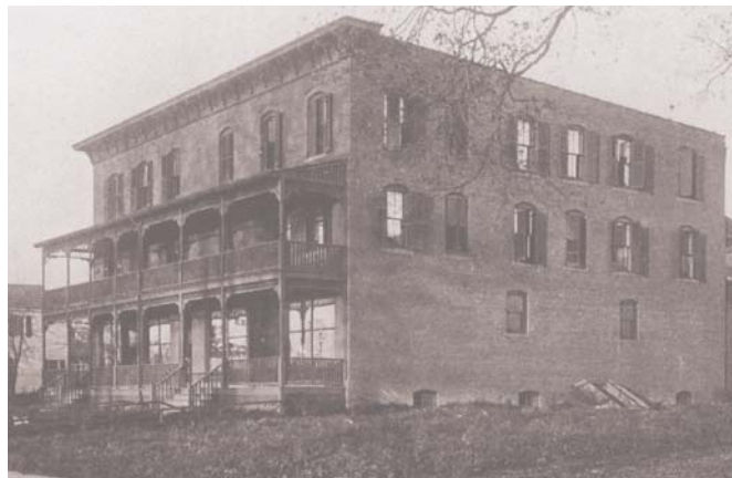
682 Wethersfield Avenue in 1899 when it housed the Industrial Home of the Connecticut Institute for the Blind. Photo: Collection of Tomas J. Nenortas
