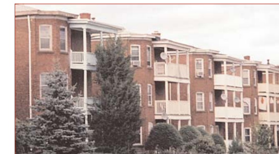
Worker housing along Capitol Avenue (left) and South Whitney Street.
