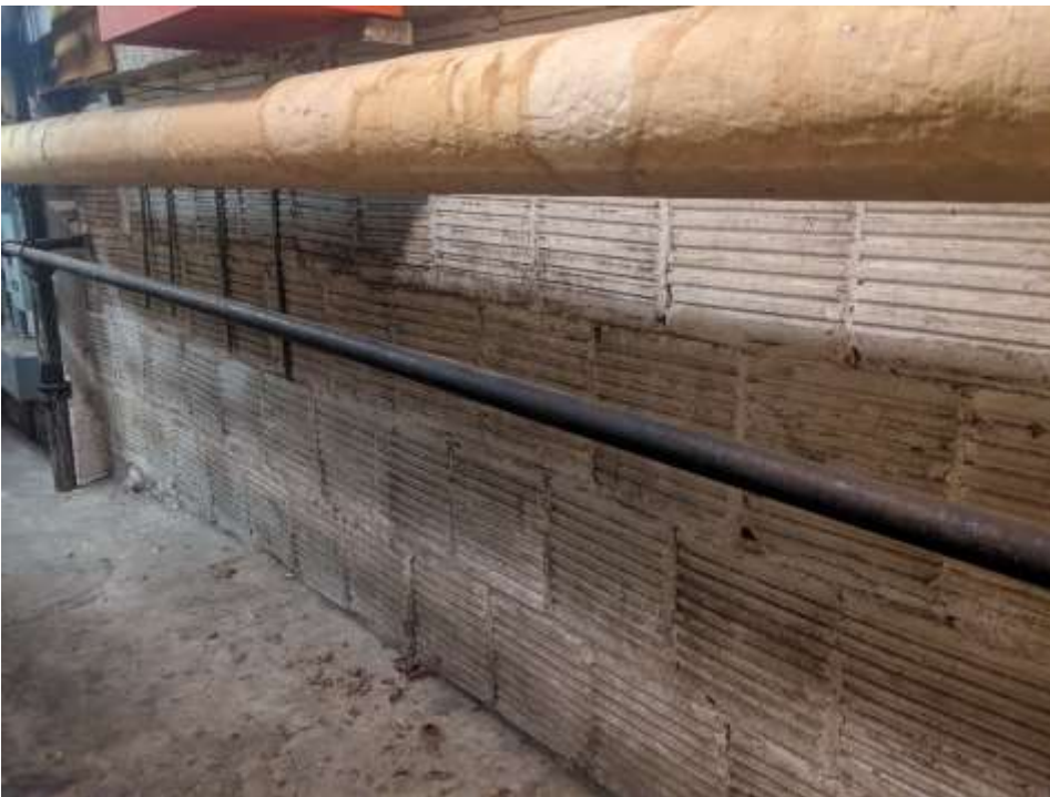
Photo 38. Example of exposed corrugated terra cotta fireproof tiling in the basement.
