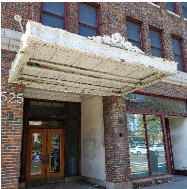
Photo 6. Main entrance with glazed mahogany doors, side lights and transoms, and marquee in center two bays of main/east elevation; at right is one of two storefronts in the northern bays.
