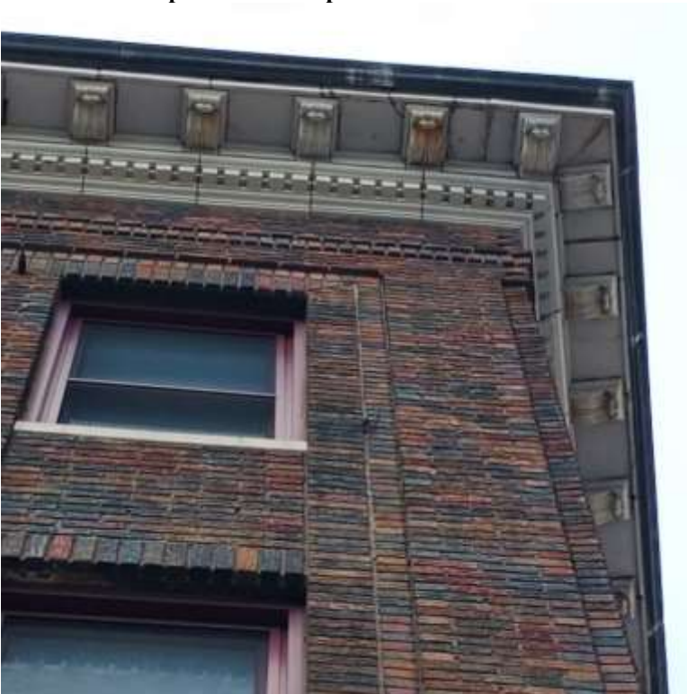
Photo 8. Close-up of projecting roof cornice; note also the brick framing of the window bay.
