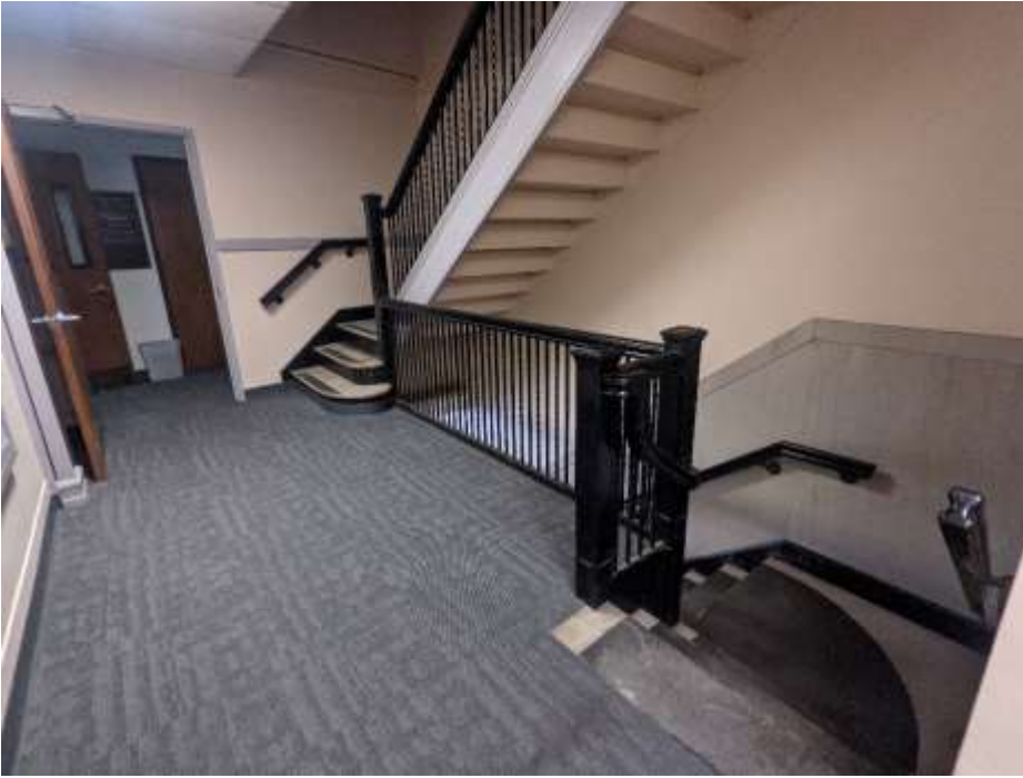
Photo 21. Second floor stairwell, landing and hall. Note the newel posts at the quarter turns, located on all levels. The marble wainscoting in the stairwell ends at the top of the first floor.
