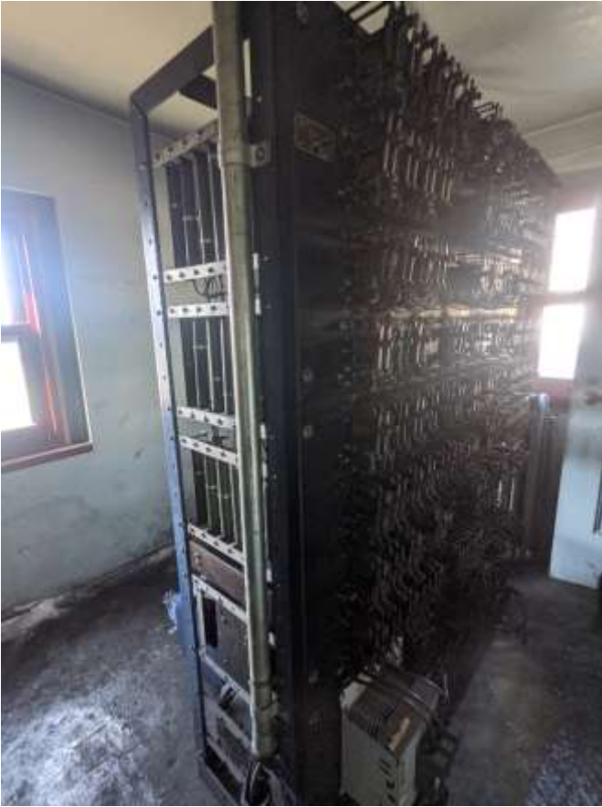
Photo 39. Elevator control panel made by F. S. Payne Co. Not shown is the adjacent elevator engine and machinery.
