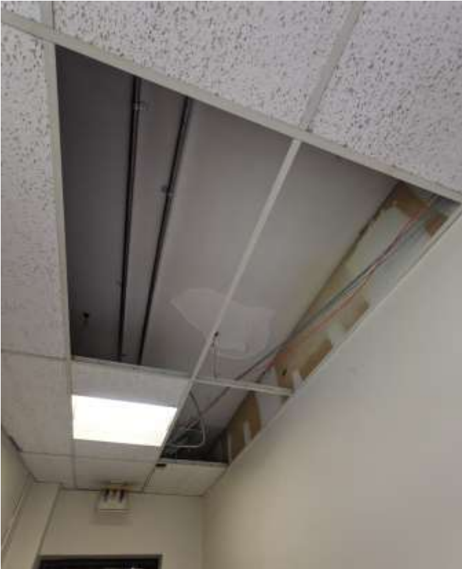
Photo 37. Exposed plaster ceiling on second floor.
