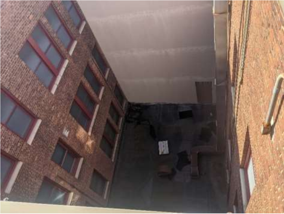
Photo 9. The well in the U looking down from the east. The concrete wall in the background was built in 1977 to close off the former staircase that became a hall with the addition of the egress tower; the first floor roof covers the original skylights.
