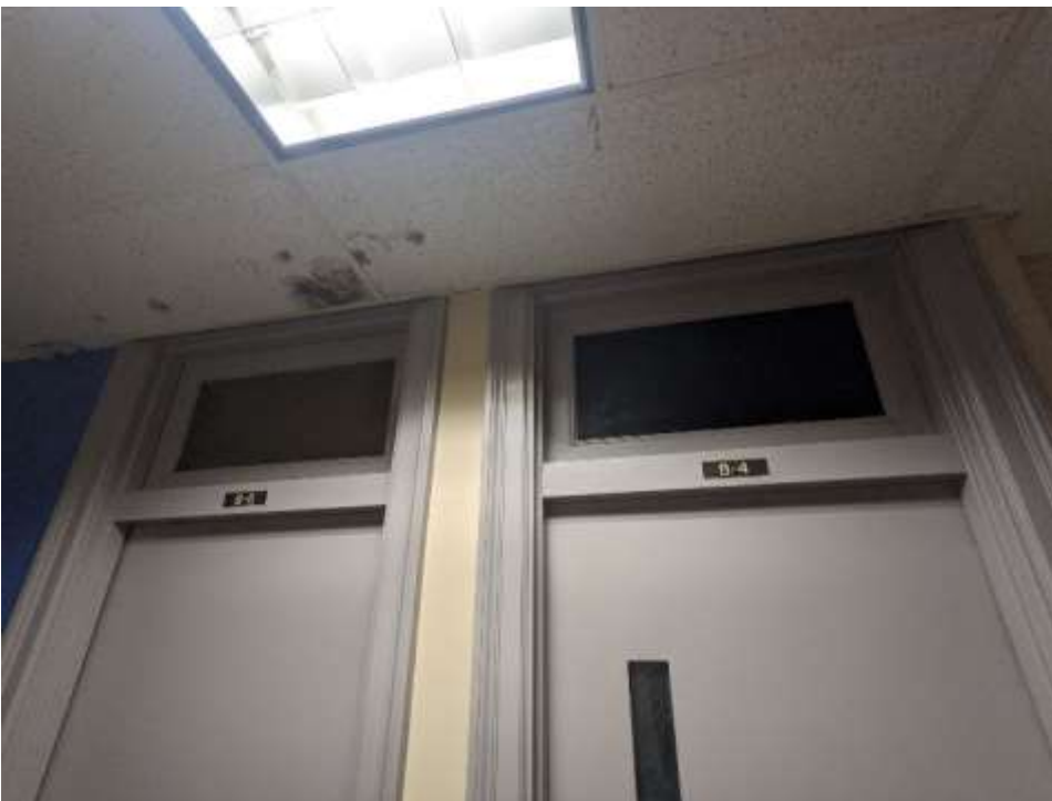
Photo 36. Surviving interior doorways with transoms at basement level; the doors themselves are replacements as the original doors were glazed.
