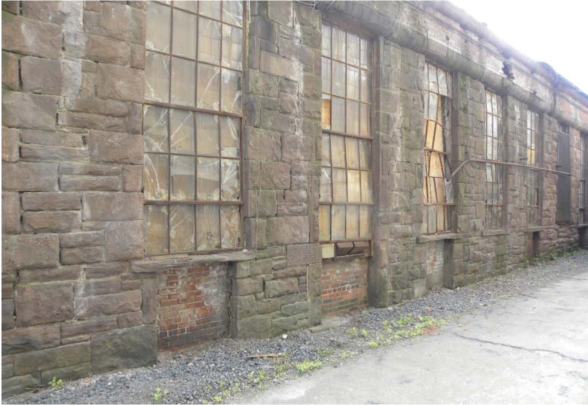
Figure 62a. Building 8, partial east elevation, looking north. The second window has been created in an original doorway as evident in the shape of the jamb units. This explains the sequence of three brick panels, instead of an alternation between brick and brownstone, below the window sills.
