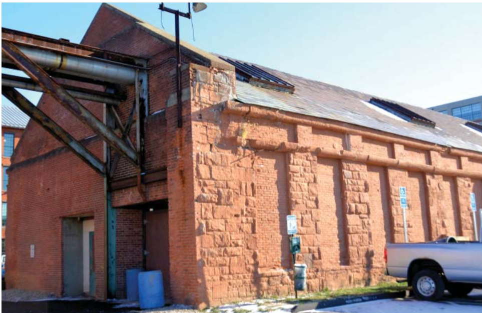
Figure 6. Building 10, northwest corner, showing brownstone architrave and cornice and brick frieze with pilasters.
