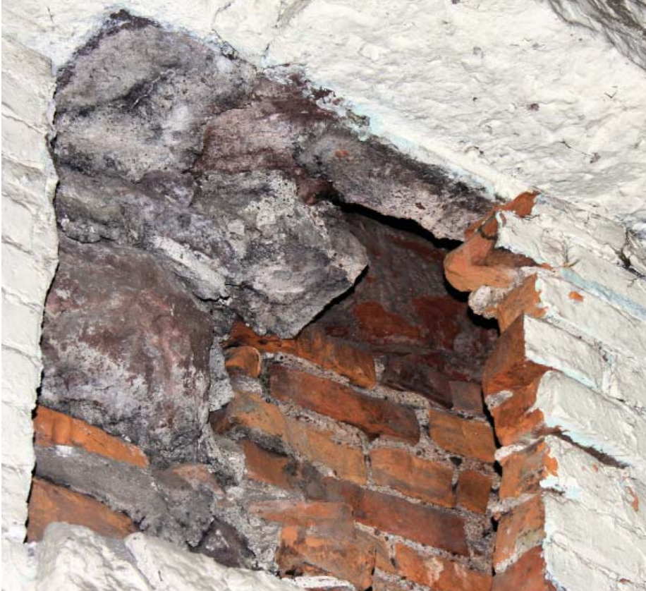
Figure 24. Opening from vertical stack to horizontal masonry duct, Building 8.
