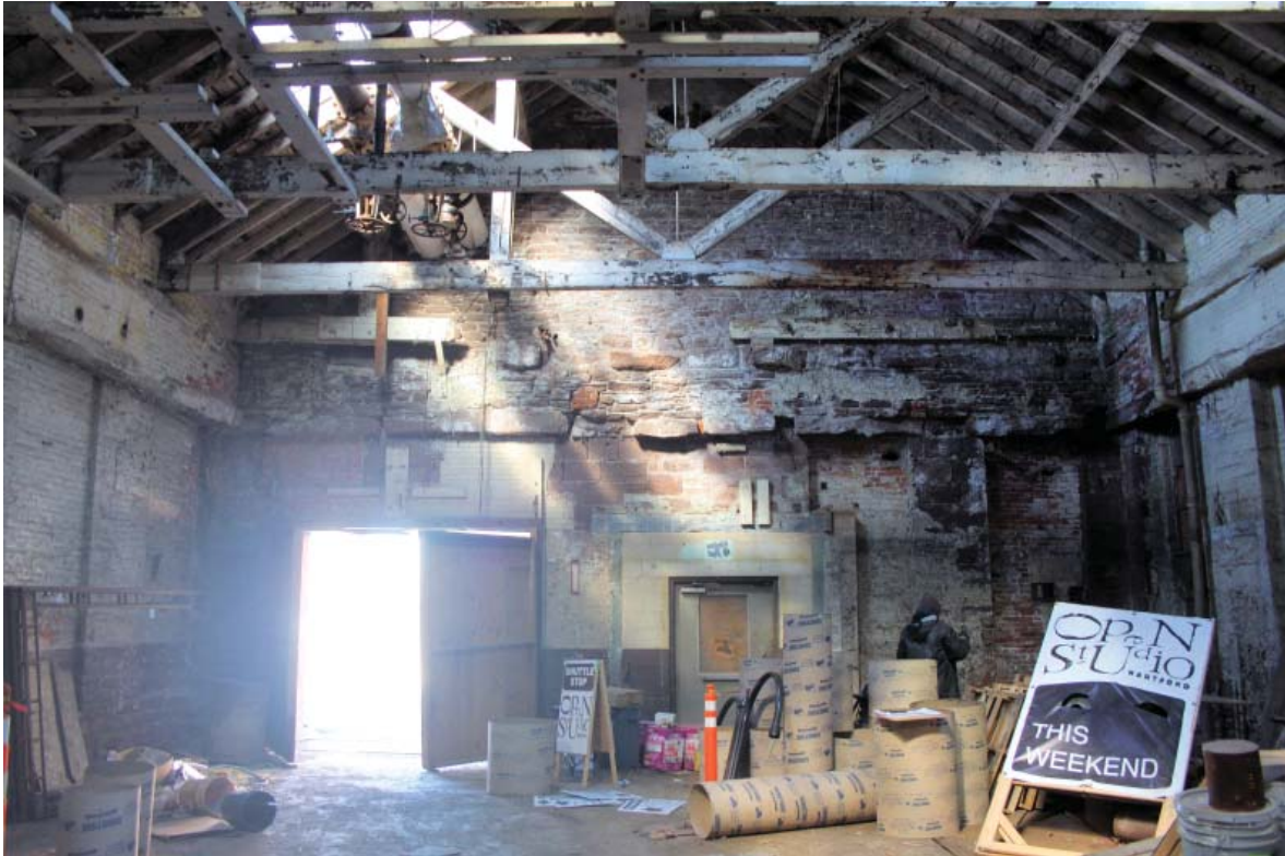
Figure 59. Building 10 as a storage facility, looking north. Note change of character due to blocked-up window openings, altered doorways, and the steam pipes overhead that served the South Armory. Brownstone units in the north wall define the course of the horizontal masonry duct in that elevation. Bricked-in window openings can be seen at the east end of the same wall.
