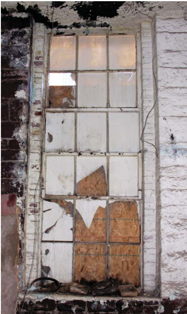
Figure 50a. Metal sash between original brick jambs, Building 10.
