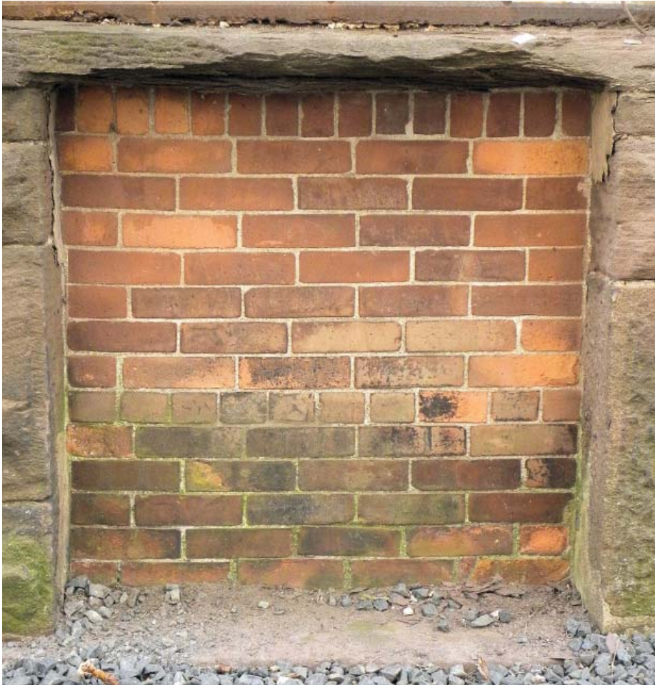
Figure 10b. Brick spandrel with sailor top course, Building 8, east elevation.
