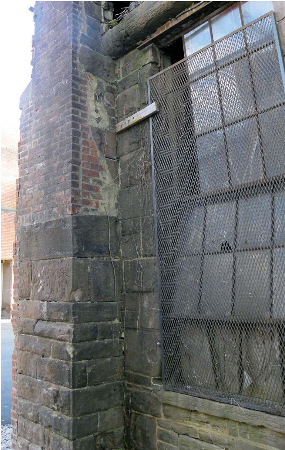
Figure 9a. Buttress, originally jamb of entry arch to passage from the north to the south court yards, Building 8, southeast corner.
