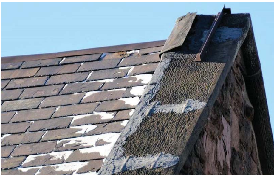
Figure 53. Metal flashing at ridge, Building 8, north end.
