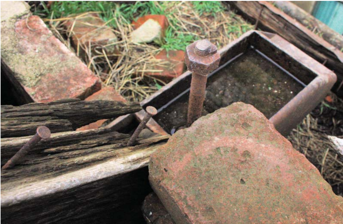
Figure 19. Cast iron shoe and anchor for truss bearing end, Building 8.
