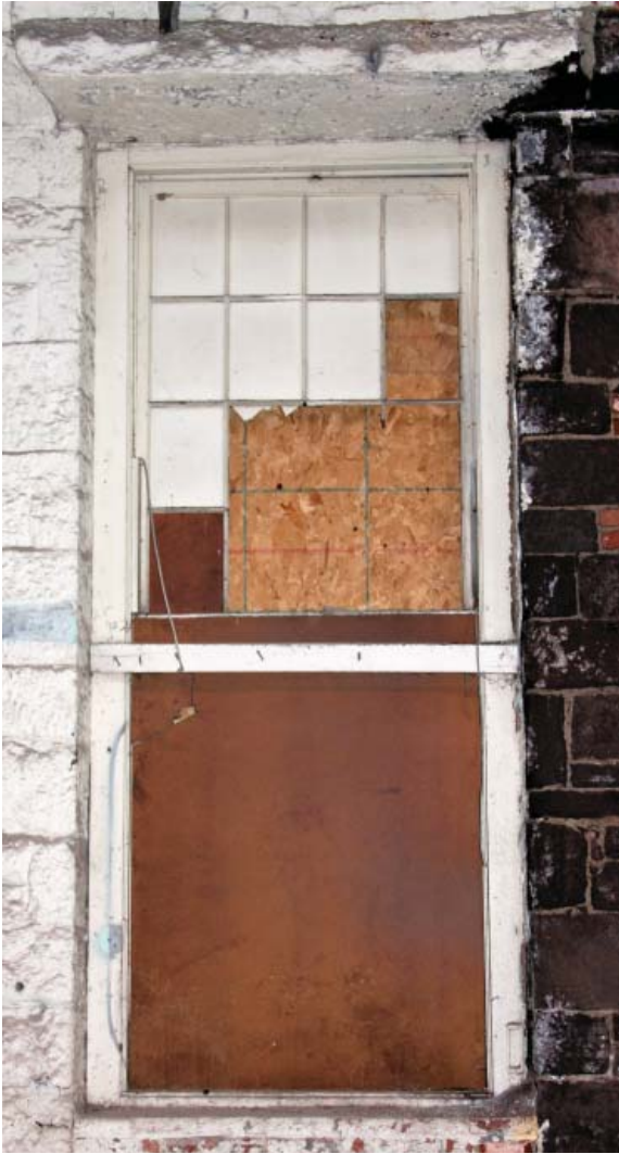
Figure 50b. Wood sash with casing over brick jambs, Building 10.
