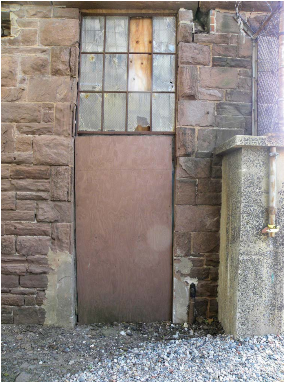
Figure 38b. Doorway created at bay 1 of east elevation of Building 8.
