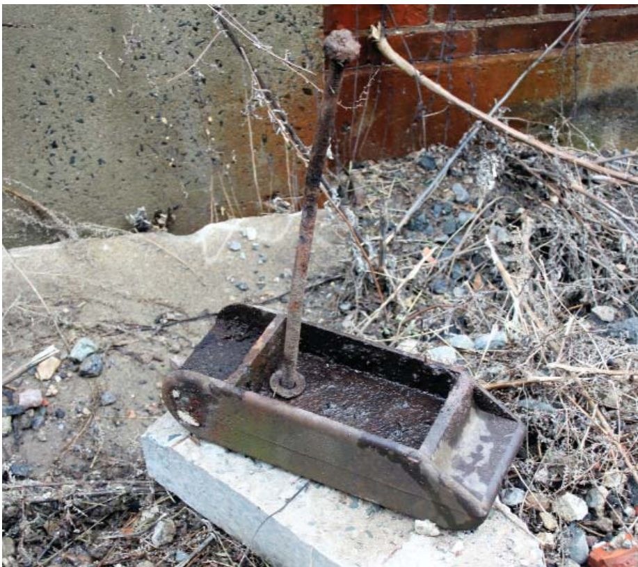
Figure 72. An unseated truss shoe.
