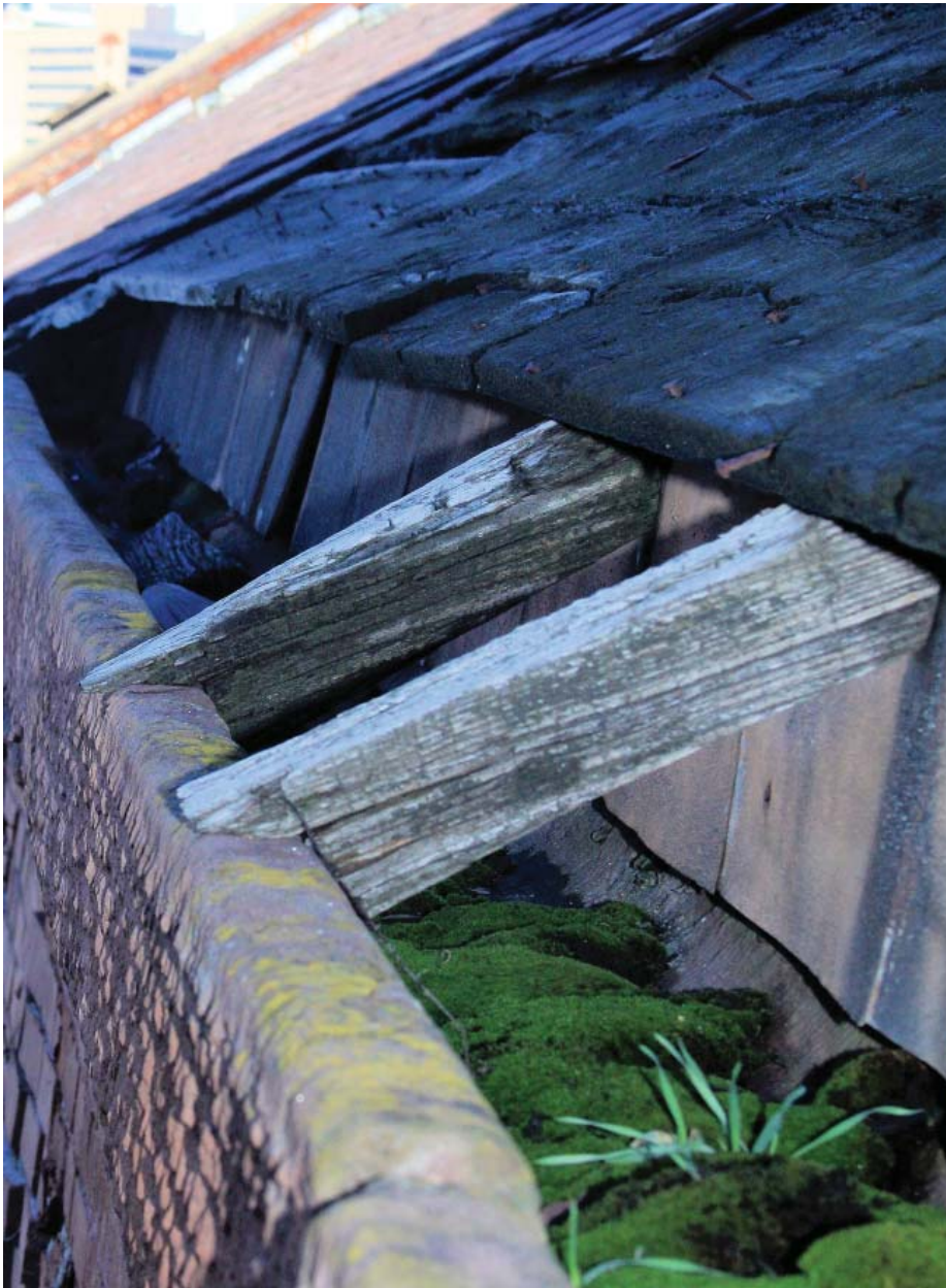
Figure 11. Kickers added over original stone gutter, Building 10, west elevation.
