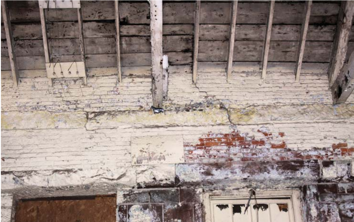
Figure 71. Representative view of upper part of interior walls, Building 10, east wall. Note remnants of an early electrical power distribution system at left.
