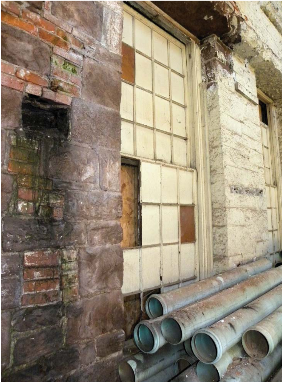
Figure 22. Typical brick patch in brownstone pier, Building 10.
