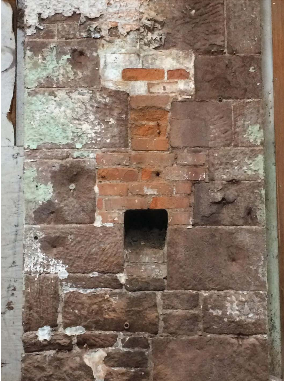
Figure 74. Building 8, interior opening to original exhaust flue shaft.
