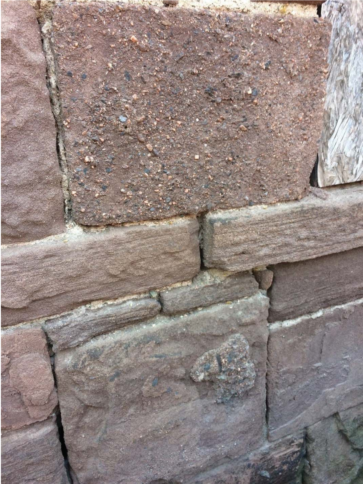
Figure 62b. Building 8, east elevation, rough aggregate concrete patches on brownstone.
