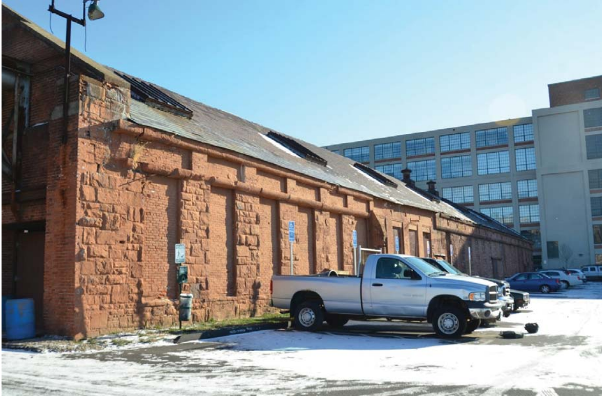
Figure 65. Building 10, west elevation. Note the brick pilasters over the brownstone piers at bays 1 through 6, bays 7 through 10 rebuilt in brick, and the open beam pockets cut into the southern stretch of the frieze.
