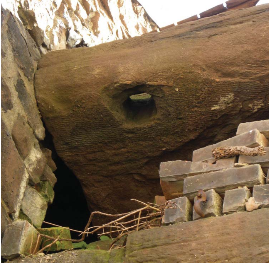
Figure 12b. Hole for outlet from stone gutter, Building 8, east bay 27.
