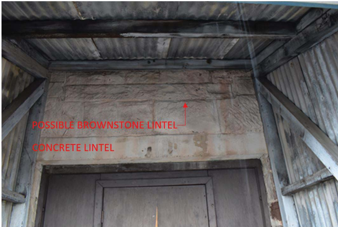
Figure 4b. Brownstone lintel set above later concrete lintel, bay W9, Building 8. Photo by J. Woolsey, NPS.
