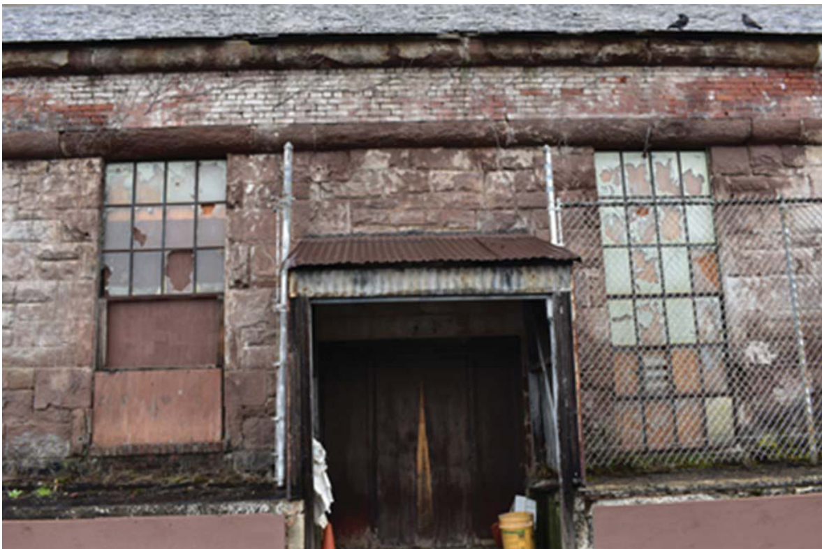
Figure 4a. Exterior of bay W9, Building 8. Note integrated brownstone masonry between the original architrave unit and the later corrugated shed roof below. Photo by J. Woolsey, NPS.
