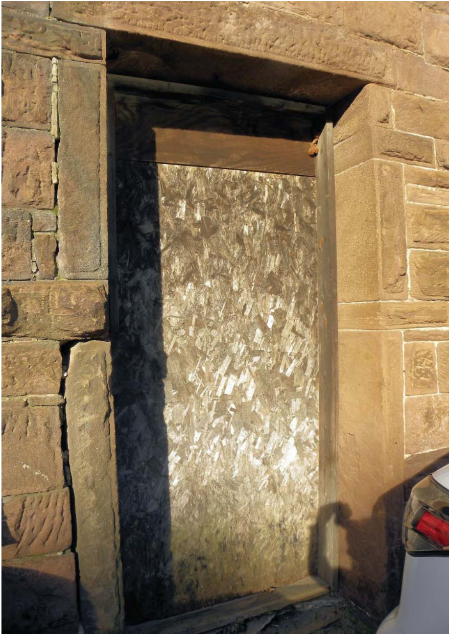
Figure 5. Typical detailing of original doorway surround, Building 10, east elevation.
