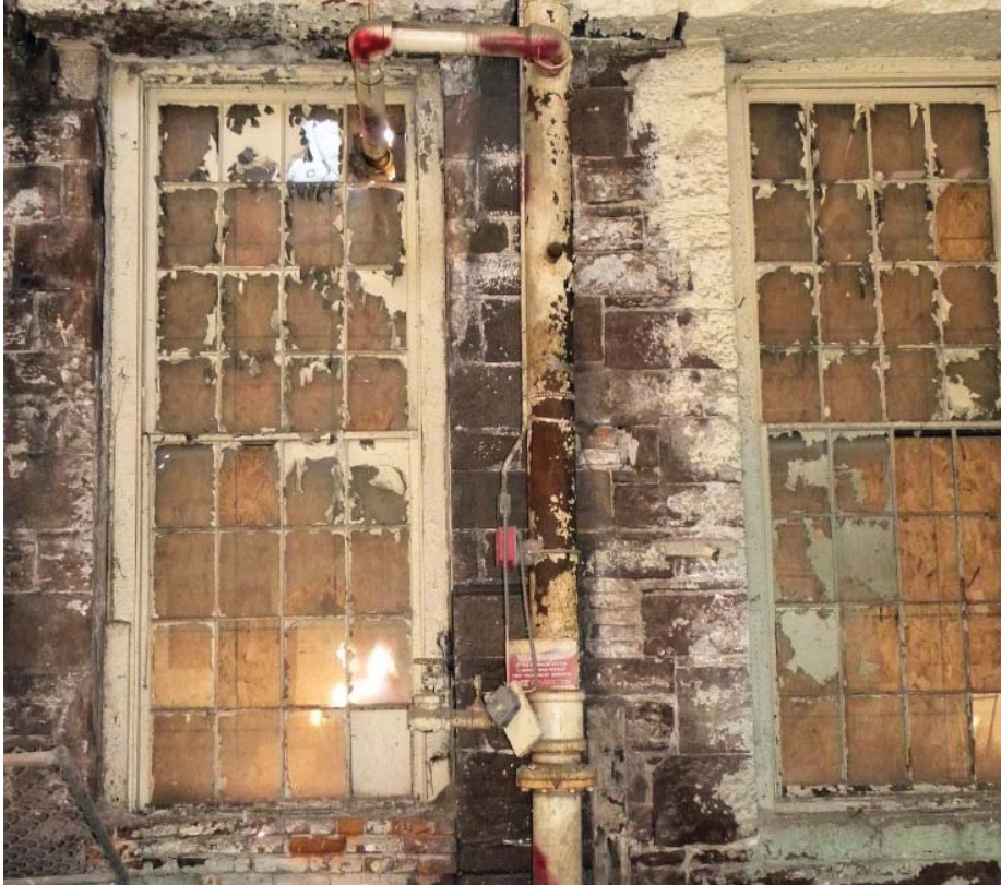
Figure 18. Characteristic view of perimeter wall bay, Building 10, east wall. Note wood windows and casing and alternating brick and brownstone masonry panels below.
