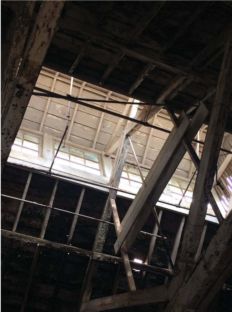
Figure 76. Building 8, central rooftop monitor.
