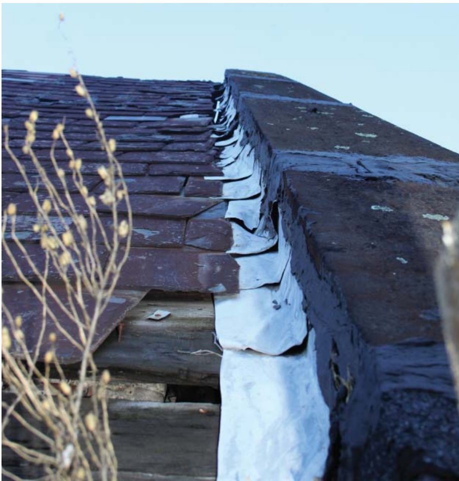
Figure 54. Lapped flashing at the south gable end of Building 10.
