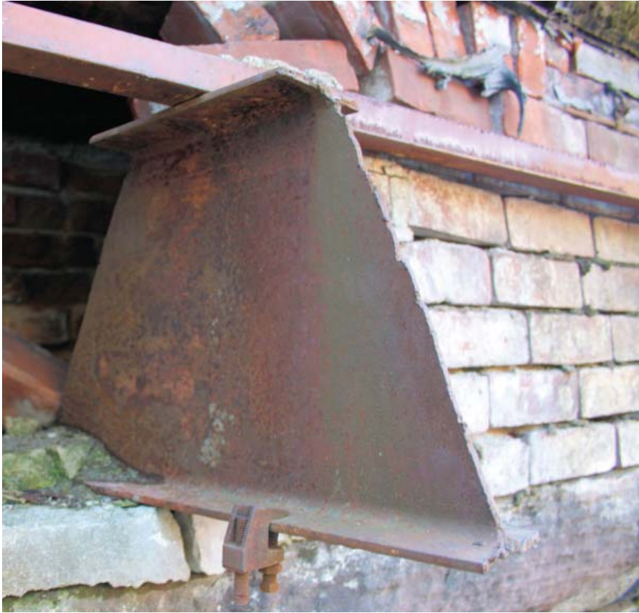
Figure 44. Typical cut end of roof beam, Building 10, east elevation.
