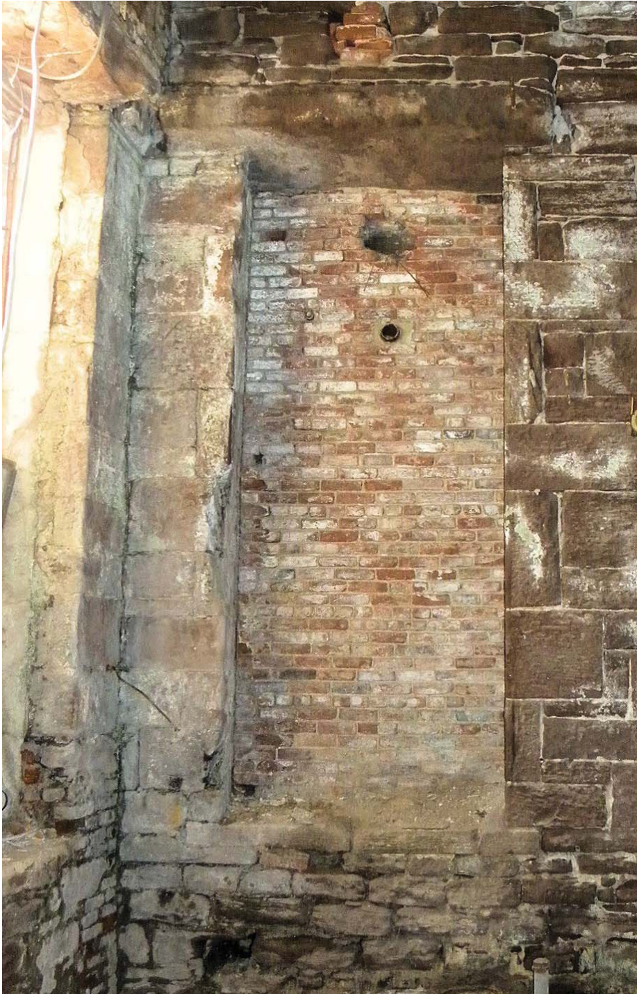
Figure 10a. Infilled window opening, Building 8, south interior elevation.
