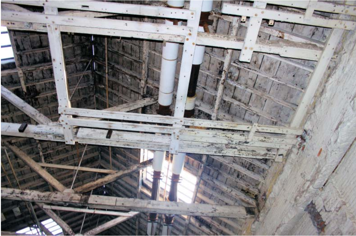
Figure 77. Skylights and steam piping at Building 10. Note daylight where ridge flashing is missing and ancillary framing below trusses.
