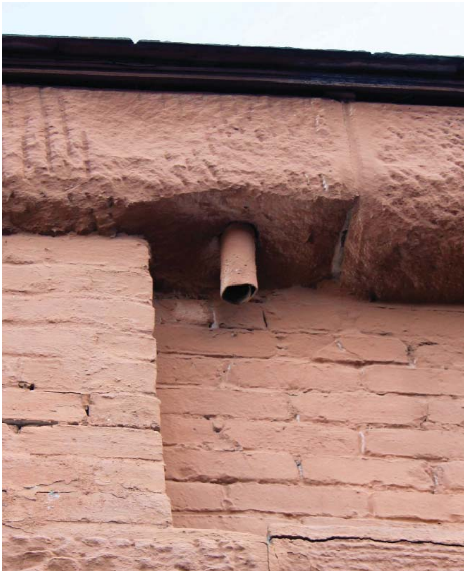
Figure 12a. Outlet from stone gutter, Building 10, west elevation.
