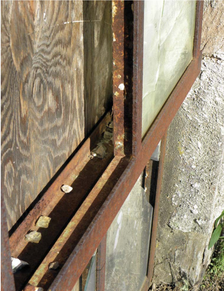
Figure 51a. Bar stock frame with ridged glass, Building 8.
