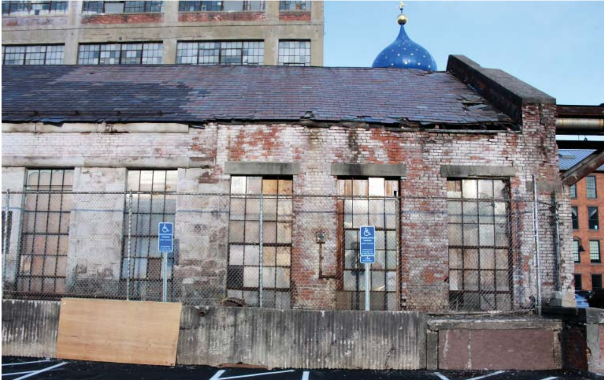
Figure 61. Mismatched slate at the south end of Building 8, west roof slope. In the foreground is the raised, early 20th century steam tunnel. The last three window bays are not original. Note missing slates at eave and water damage to masonry below.
