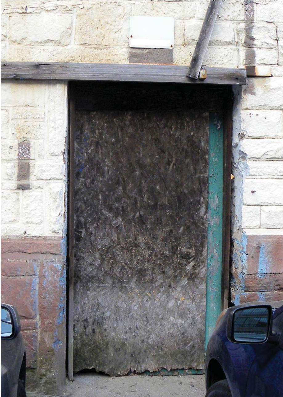
Figure 45a. Enlarged exit doorway cut into original door opening, bay 19, Building 10, east elevation.
