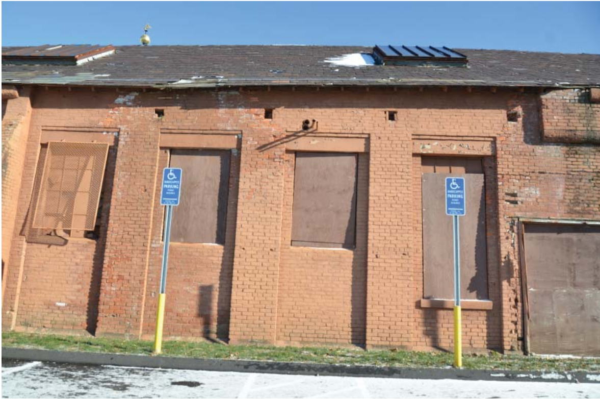
Figure 42a. Brick reconstruction of bays 7 through 10, Building 10, west elevation.
