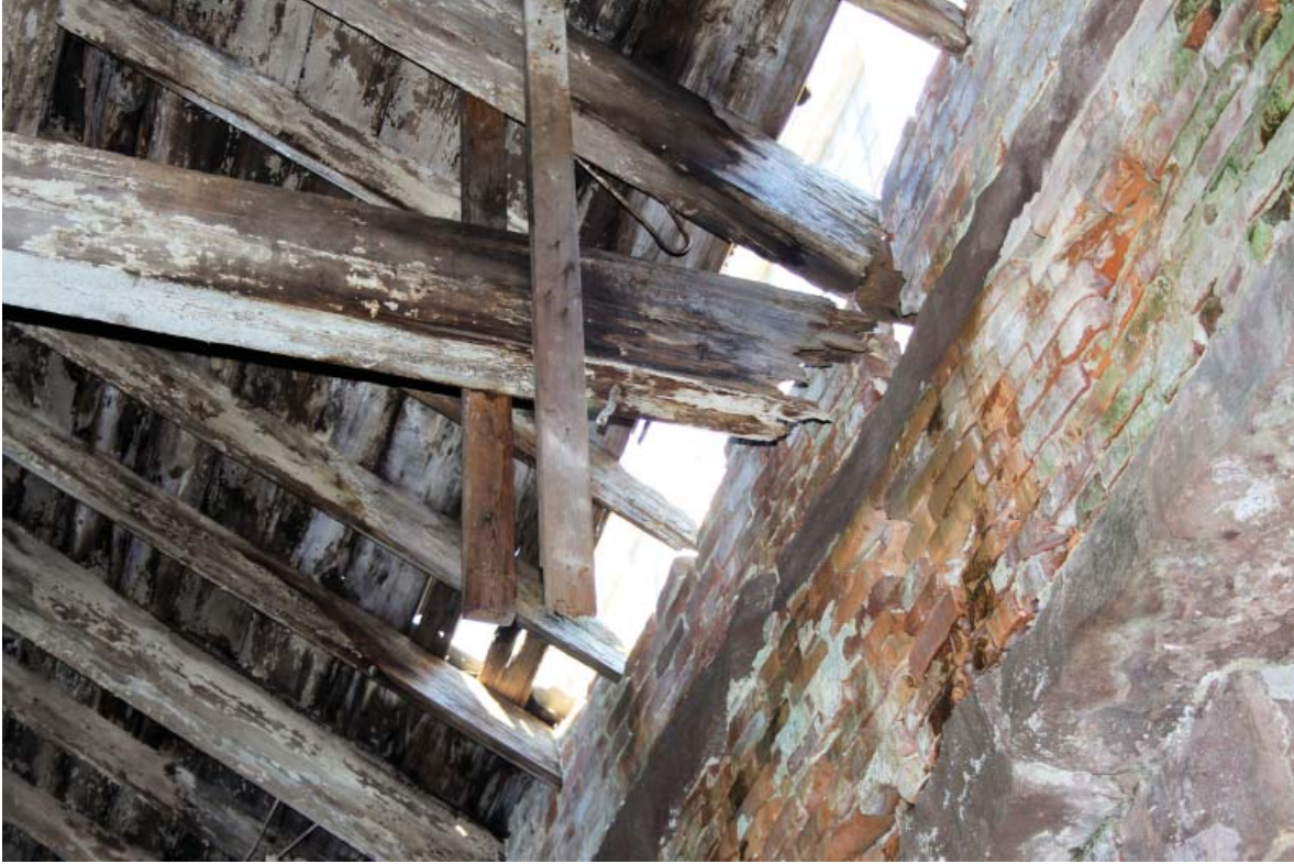
Figure 75. Missing roofing boards, east elevation, Building 8. Note metal straps joining the decayed truss elements.
