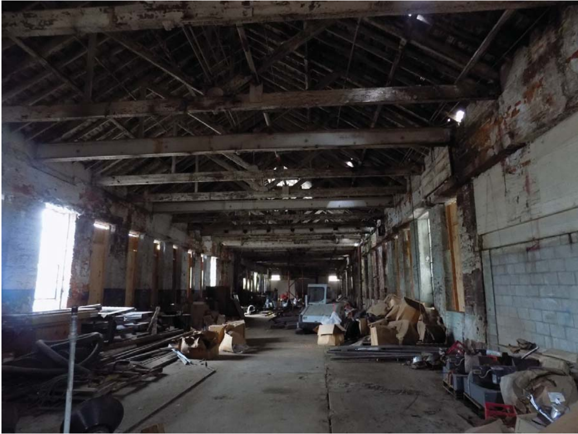
Figure 70. Scaffold support, Building 8, interior looking north. Note concrete block infill of later doorway at bays 19 & 20 at right.
