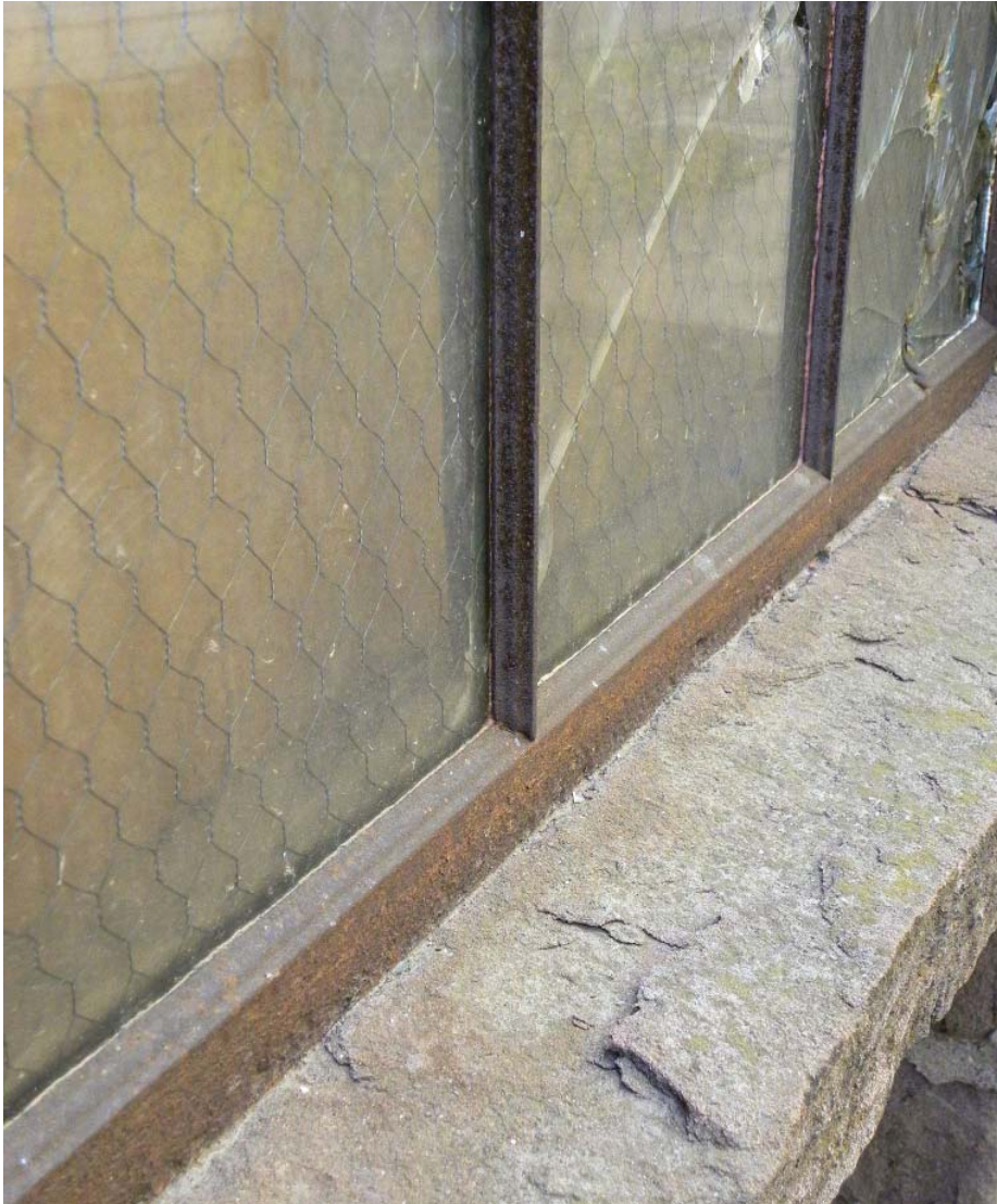
Figure 51b. Profiled metal frame with wired glass, Building 8.
