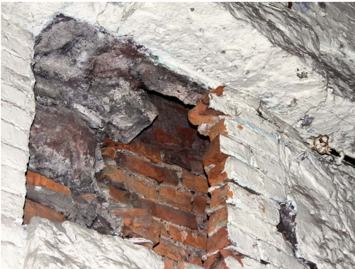
Figure 73. Masonry shaft with opening into masonry duct above.
