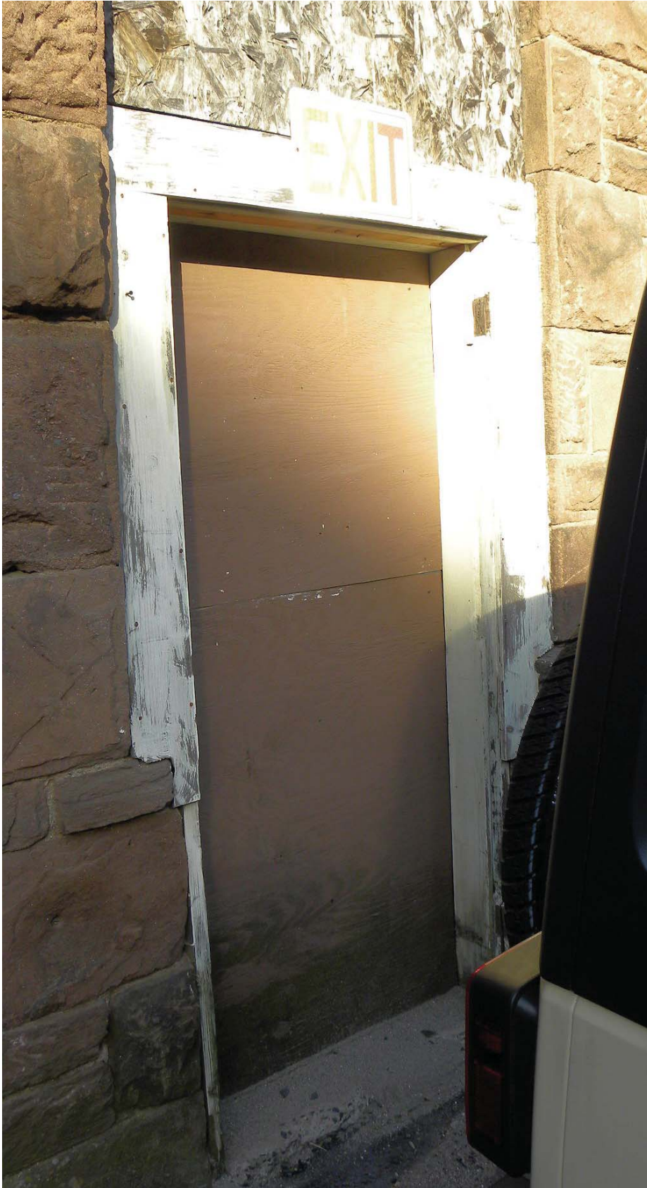
Figure 45b. Doorway cut into window bay 12, Building 10, east elevation.
