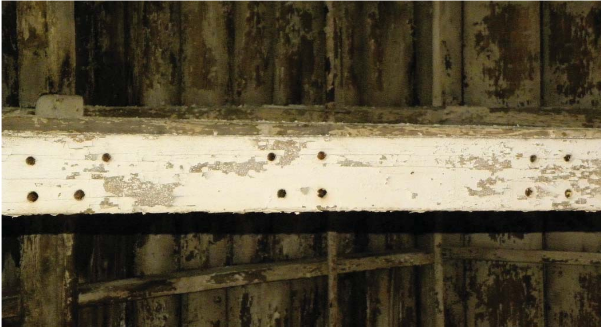
Figure 25. Representative pattern of holes in bottom chord of a truss, Building 8.
