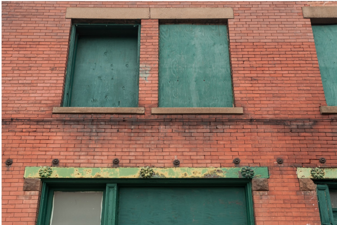
Photo 3. Mansuy and Smith Automobile Showroom Building, view north showing Iron lintels, rusicated brownstone blocks, Iron rosettes and second story windows..
