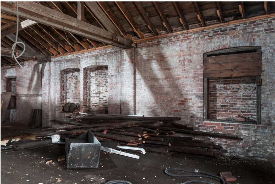
Photo 16. Mansuy and Smith Automobile Showroom Building, second story, view southwest showing bricked-in window openings.
