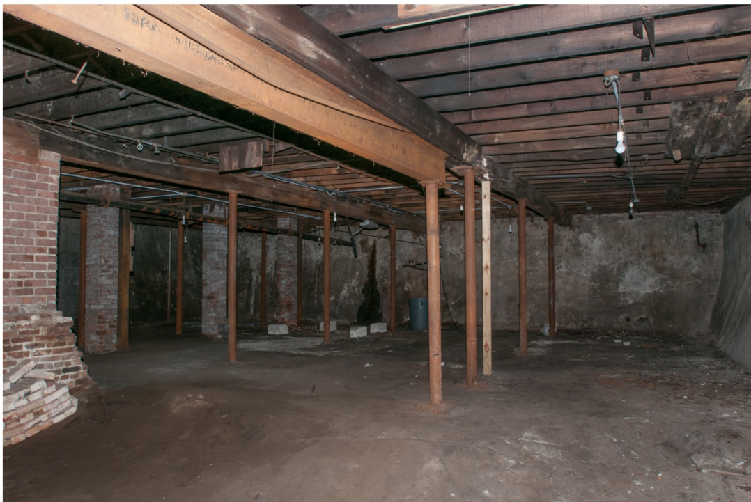
Photo 18. Mansuy and Smith Automobile Showroom Building, basement, view southeast showing stone foundation, floor joists, brick columns, round steel columns and part of partial wall.
