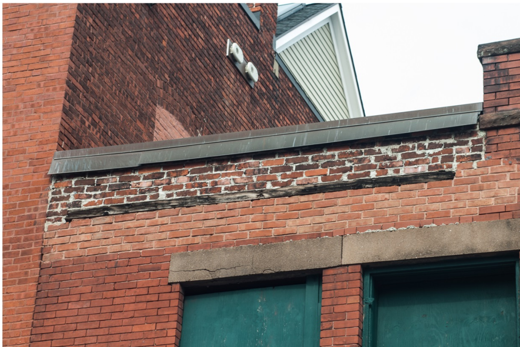
Photo 4. Mansuy and Smith Automobile Showroom Building, view north showing repairs to west bay cornice.
