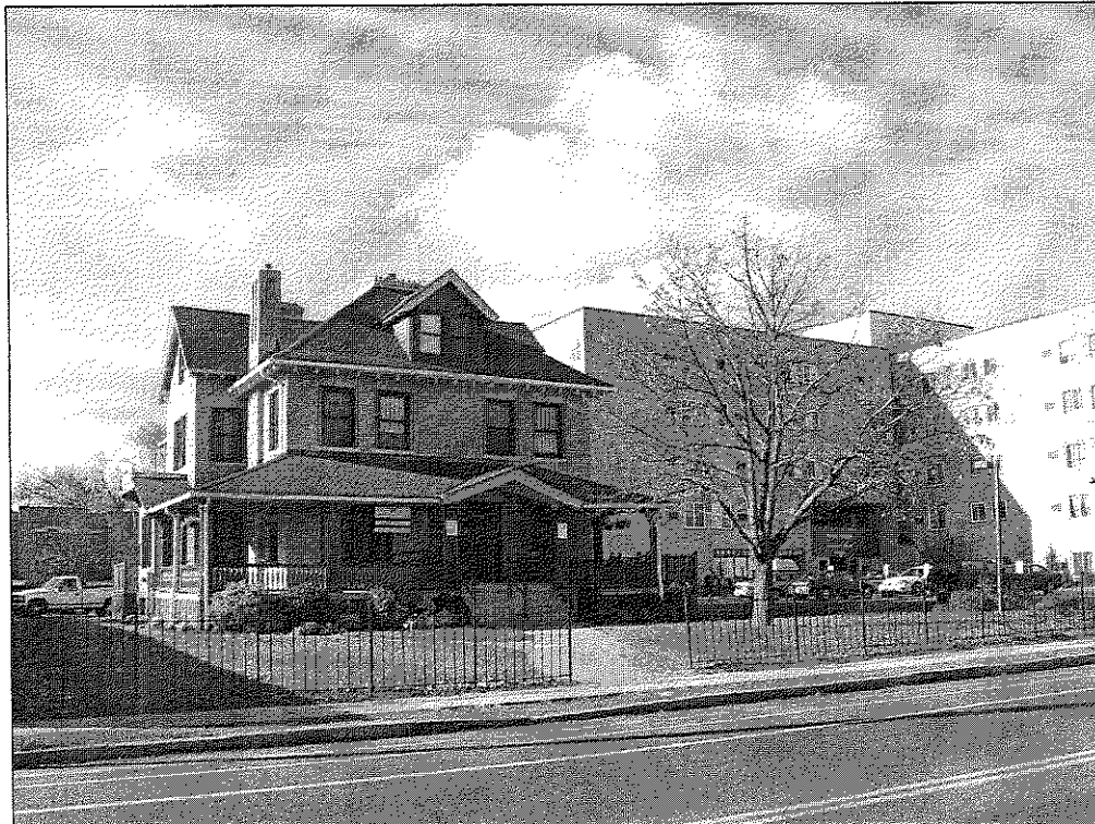
Photo 16: View looking northwest from Vine St. between Albany Ave. & Mather St.
