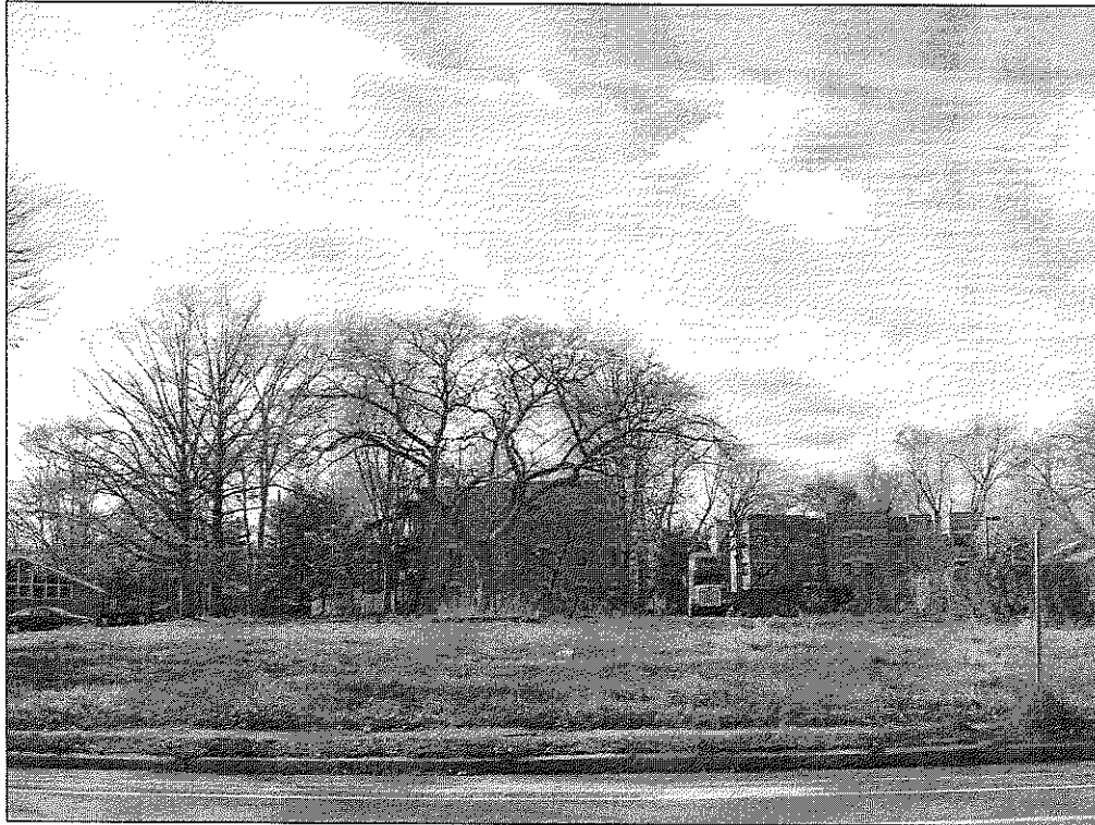
Photo 17: View looking west from Vine St. between Albany Ave. & Mather St.
