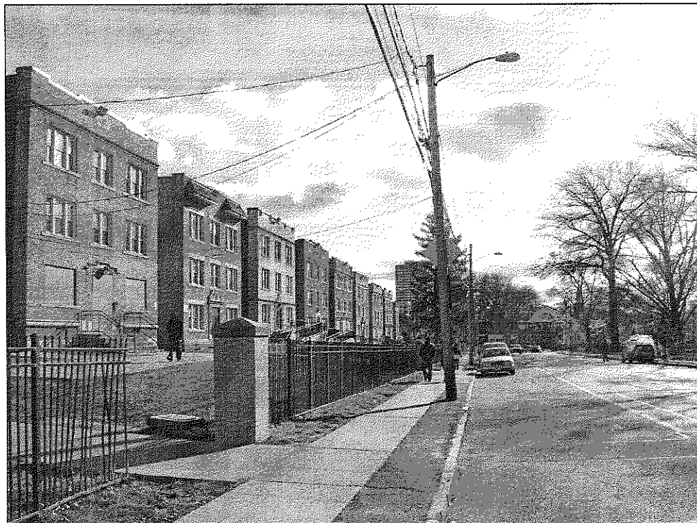
Photo 02: View of Vine St. apartments blocks, Hartford, looking southwest (left to right: #32-24, #28-30, #24-26, #22-20, #16-18, 12-14, 8-10, #4-6)
