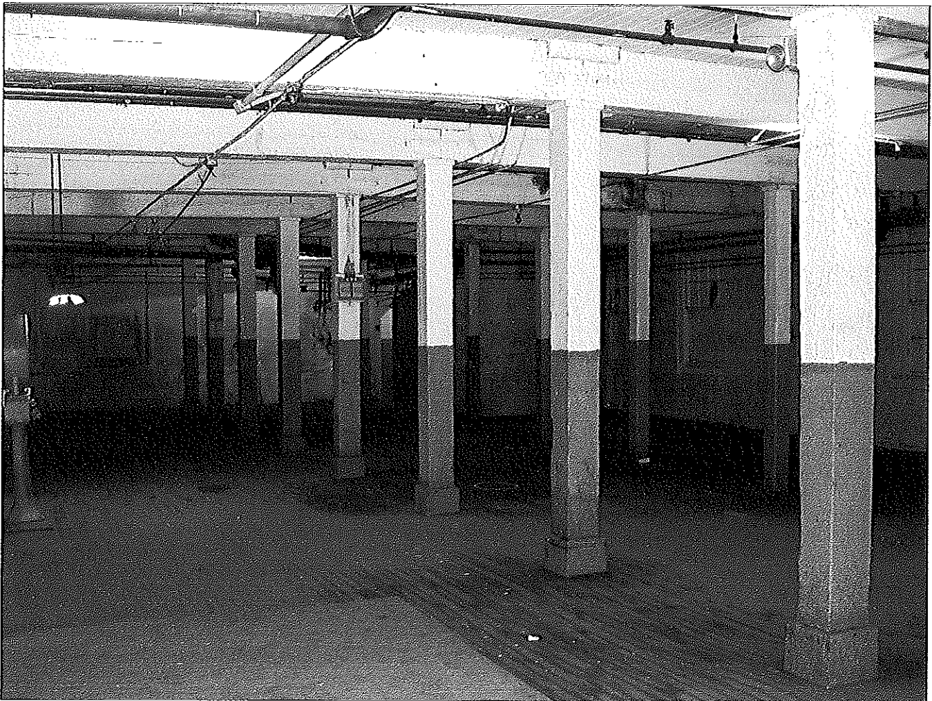
Photograph 9: Typical interior framing of timber columns and beams.
