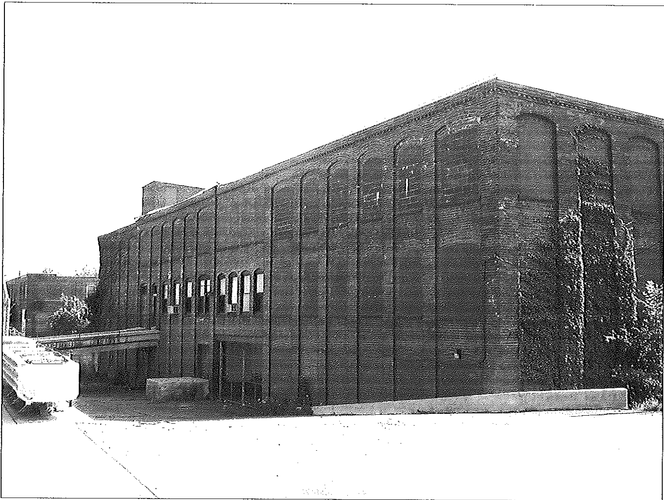
Photograph 1: West elevation, facing Woodland Street, camera facing northeast. The main entrance was via the bridge to the central portion's second story.
