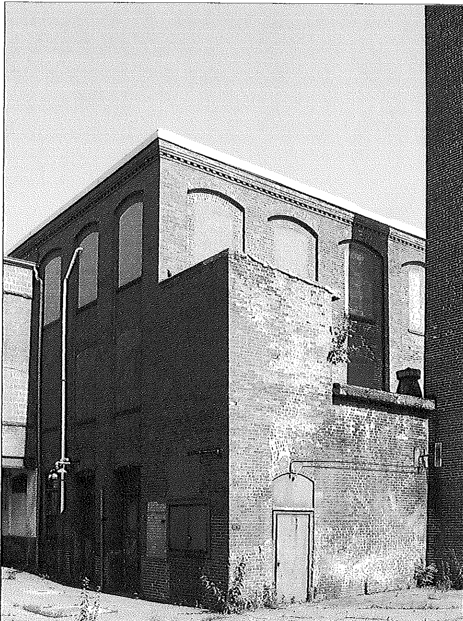
Photograph 5: Boiler house at rear of original factory, camera facing northwest.
